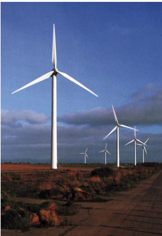
Figure 1: Wind power generators are now common worldwide. Great Orton Windcluster ©Wind Prospect / Cumbria Wind Farm
