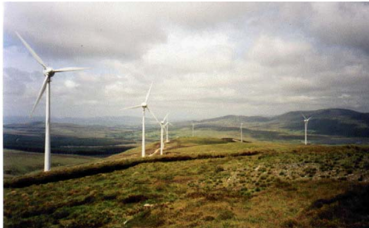
Figure 3: Crockahenny Windcluster with installed capacity of 5 MW supplying 4200 homes ©Wind Prospect
