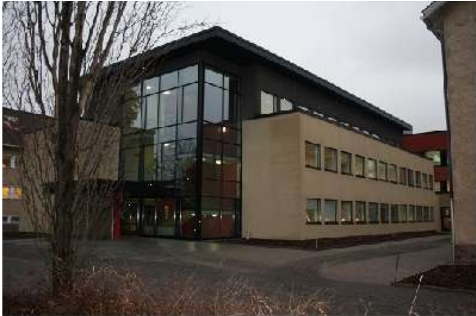
FIGURE 21. X-building of University of Applied Sciences in Mikkeli, Finland
