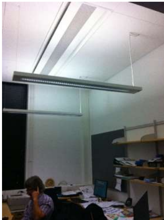
FIGURE 18. Office room in Mikpoli-building
