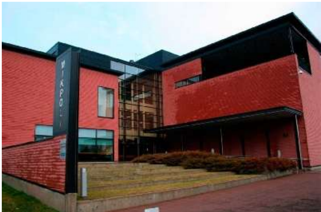
FIGURE 17. Mikpoli-building of University of Applied Sciences in Mikkeli, Finland
