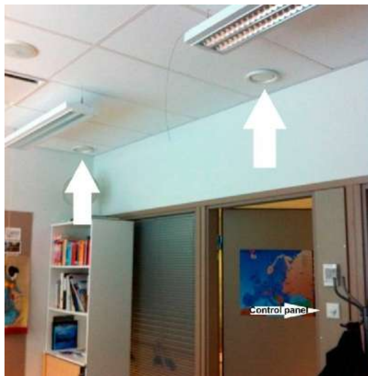
FIGURE 23. Office room in X-building
