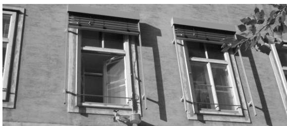
Figure 2: Windows and shades of R3
