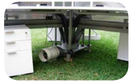
Figure 7 This system uses a ducted system distinct from the workstation
