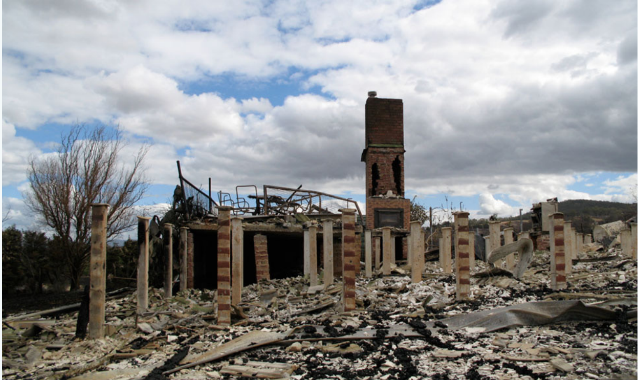
Figure 3: Yarra Glen house destroyed in the Victorian bushfires of February 2009 (Image: Wikimedia Commons)
