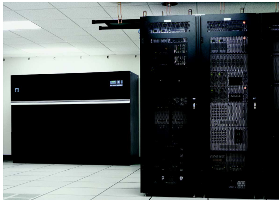
Figure 4. Precision air conditioning systems are available in a range of configurations to provide room-level and rack-level protection.
